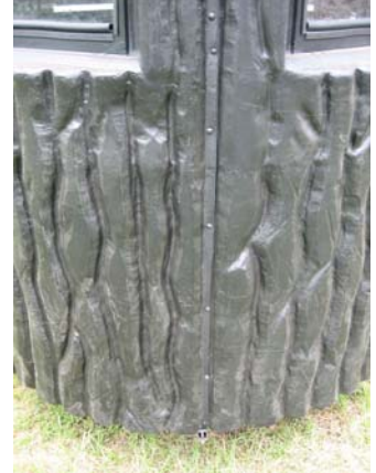
11. Drill and screw the remainder of the seams together at the dimple locations starting at the bottom and working up. Repeat with 3rd panel.
