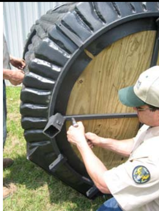
27. Tighten floor bolts with 9/16" socket wrench.
