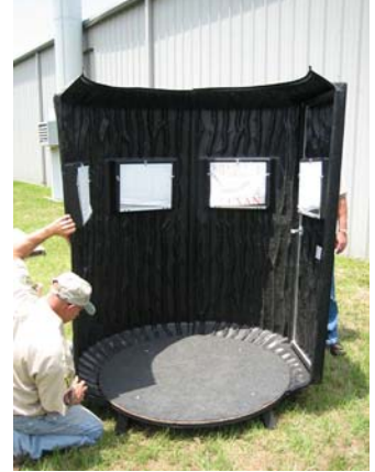
5. Install a second panel between floor and ring same as door panel.
