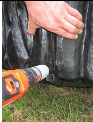
6. Overlap 1" wide seams. Locate bottom dimple in seam for screw location. Drill with 1/8" drill bit.
