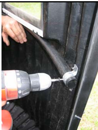
16. Pipe ring should extend past clamp about 1/2". Fasten with #2 x 1/2" self drill screw through center of clamp in to pipe ring.
