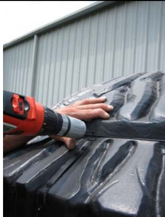
24. Align a dimple in top lip with side seam. Drill with 1/8" bit and fasten with #8-32 x 3/4" SEM screw & speed nut. Repeat at all dimple locations.
