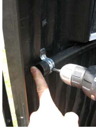
22. While slightly pushing on end of pipe to eliminate any slack, fasten end of pipe through clamp with #2 x 1/2" self drill screw to hold in place.
