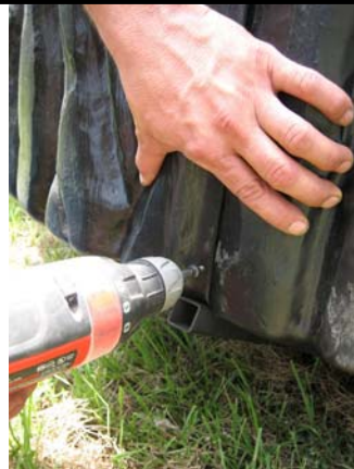
7. Use Phillips head driver to run #8-32 x 3/4" SEM screw through drilled holes.
