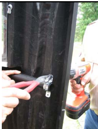
15. Fasten clamp with 2 #8-32 x 3/4" SEM screws and speed nuts.
