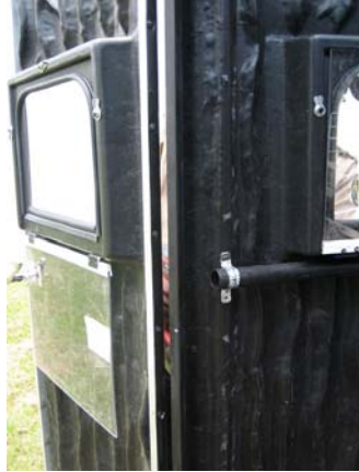
21. Double clamp should be located in recess to the right of door and fastened with pipe level with bottom of window.
