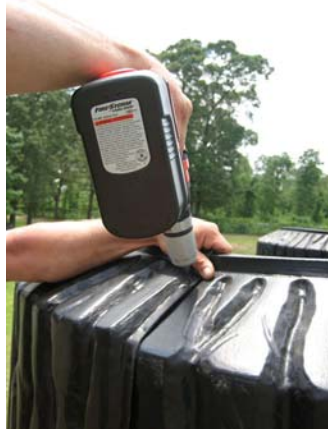
9. Align seams at top of panel & drill.
