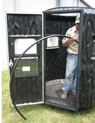
12. Install center support 1" pipe ring.
