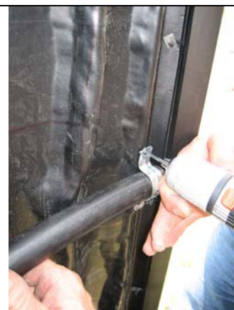
14. Drill clamp holes from inside with 1/8" drill bit.
