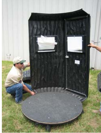
3. Insert bottom lip of blind between 1/2" plywood floor & tower ring.
