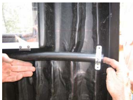
13. Start at the left hand side of door facing outward. Align ring with bottom of adjacent window. Place double clamp in recessed area over end of pipe ring.
