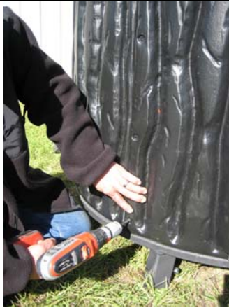
7. Overlap panels as shown and insert 3/4" SEM screw starting at bottom position first.
